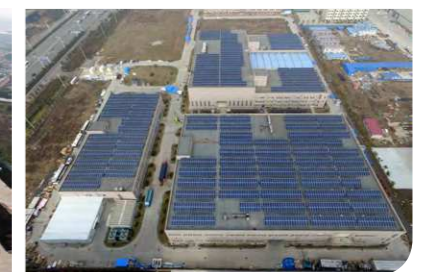
晶澳合肥通彩分布式电站 JA Solar's Tonsail Distributed Photovoltaic Power Plant in Hefei
