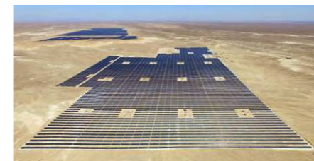
晶澳新疆和丰30MW光伏电站 JA Solar's 30MW Photovoltaic Power Plant in Hefeng, Xinjiang
