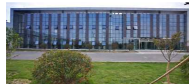
扬州基地BIPV项目 BIPV Project in Yangzhou Manufacturing Base
