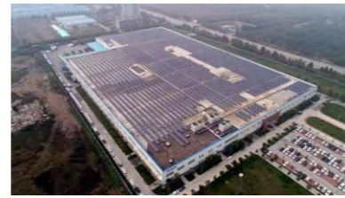
邢台基地厂房分布式项目 Plant Distributed Project in Xingtai Manufacturing Base
